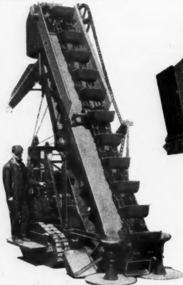
The new Barber-Greene "25," for short run and lighter work. Capacity: more than one cubic yard of loose material per minute.
